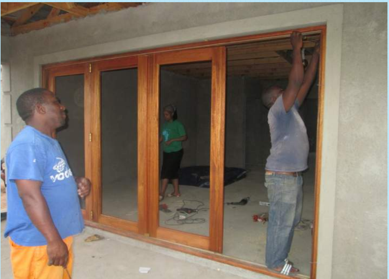
Maczen technicians on site installing wooden sliding door
