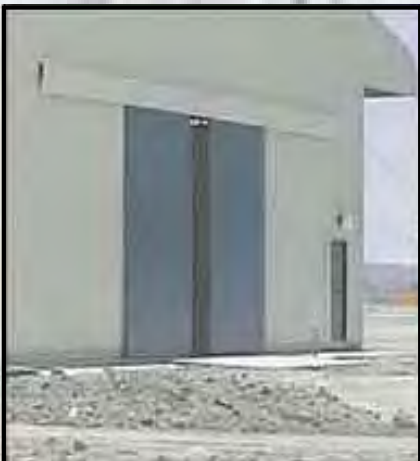
Bi-parting top hung Q-deck door installed at Impala platinum park
